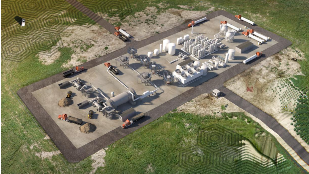
Image of Raven SR's Facility
